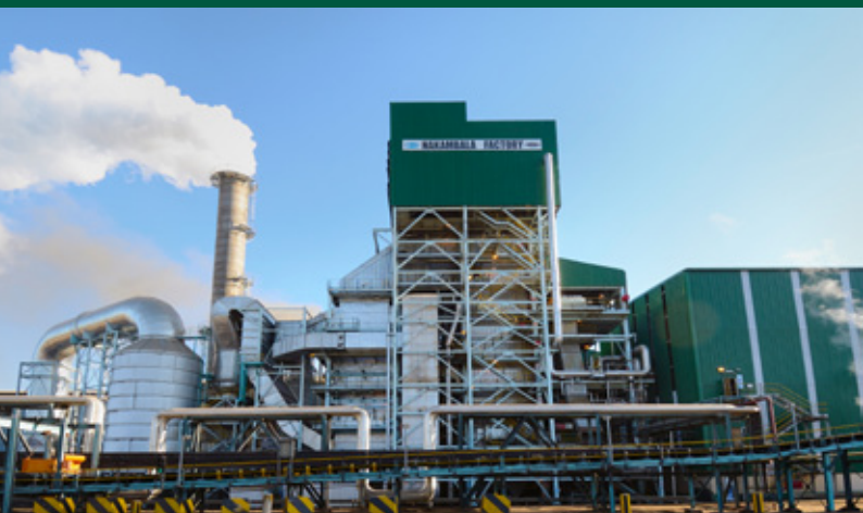
The expanded Nakambala factory. Record sugar production of 404 000 tons was achieved compared to 374 000 tons in the previous season.
