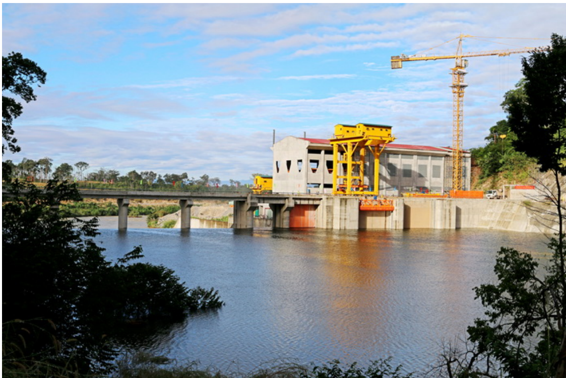
XEKAMAN XANXAY hydropower plant
