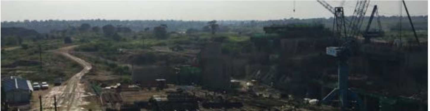
Isimba Hydroelectric Power Station construction site, Uganda. 2016
