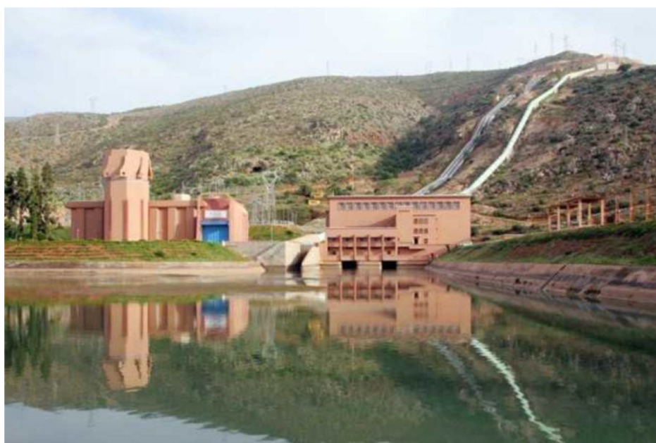
Fig. 6. Hydroelectric Plant near Agadir – Morocco [42].
