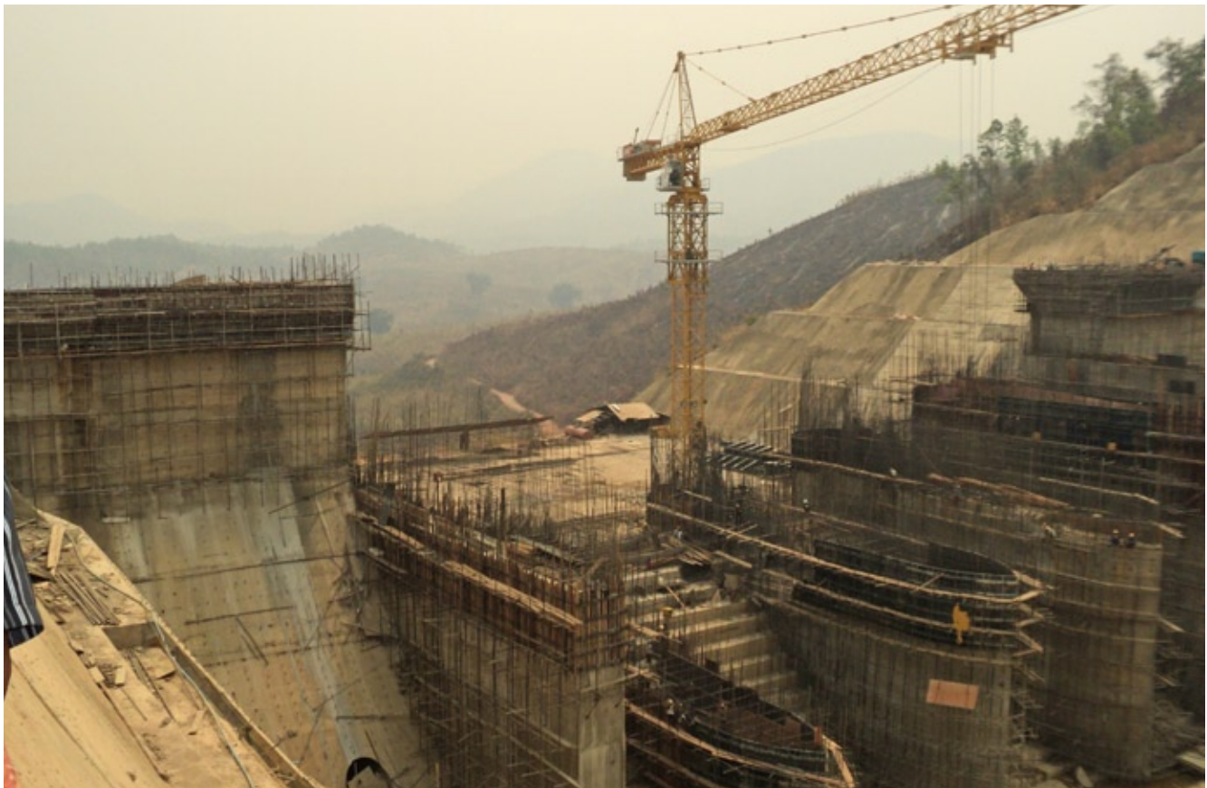
Construction of Thaukyekhat-2 hydropower dam near Toungoo in Karen State (KESAN)
