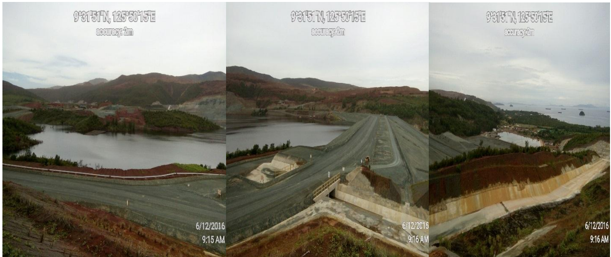
Geotagged photo of Tailings Storage Facility
