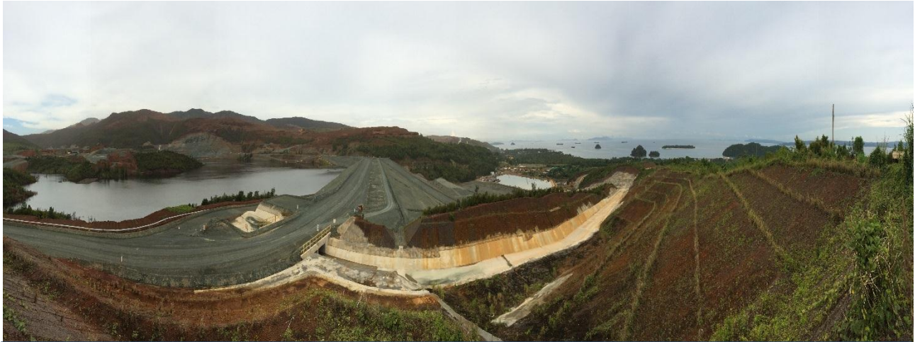
Panoramic view of Tailings Storage Facility
