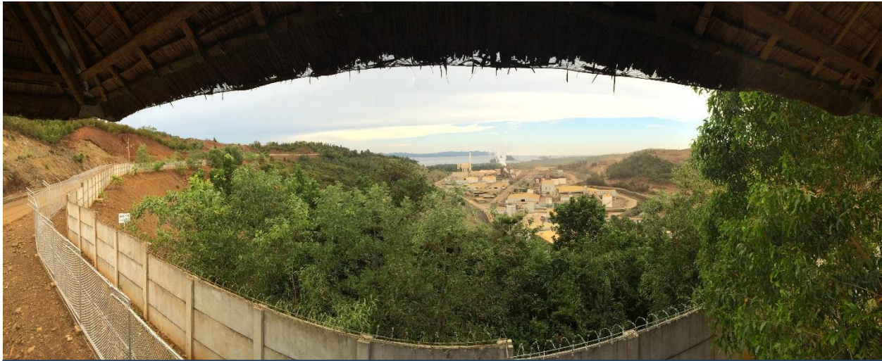
Panoramic view of Taganito Hydrometallurgical Processing Plant Complex
