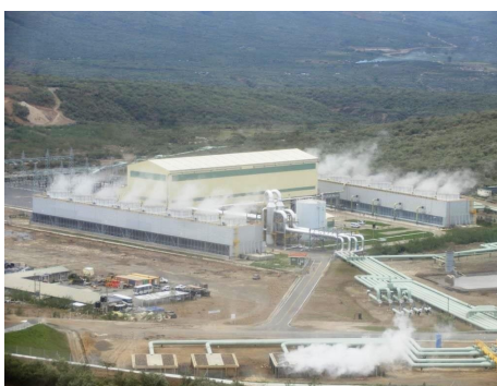
Olkaria IV Geothermal Power Plant
