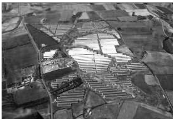
Photo: Enervitabio Ltd Santa Reparata, solar greenhouses, Narbolia
