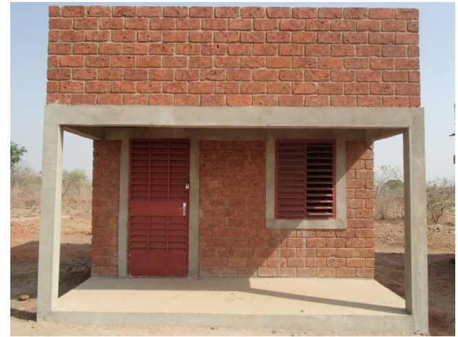
New houses built for resettlement program (400 houses to build)
