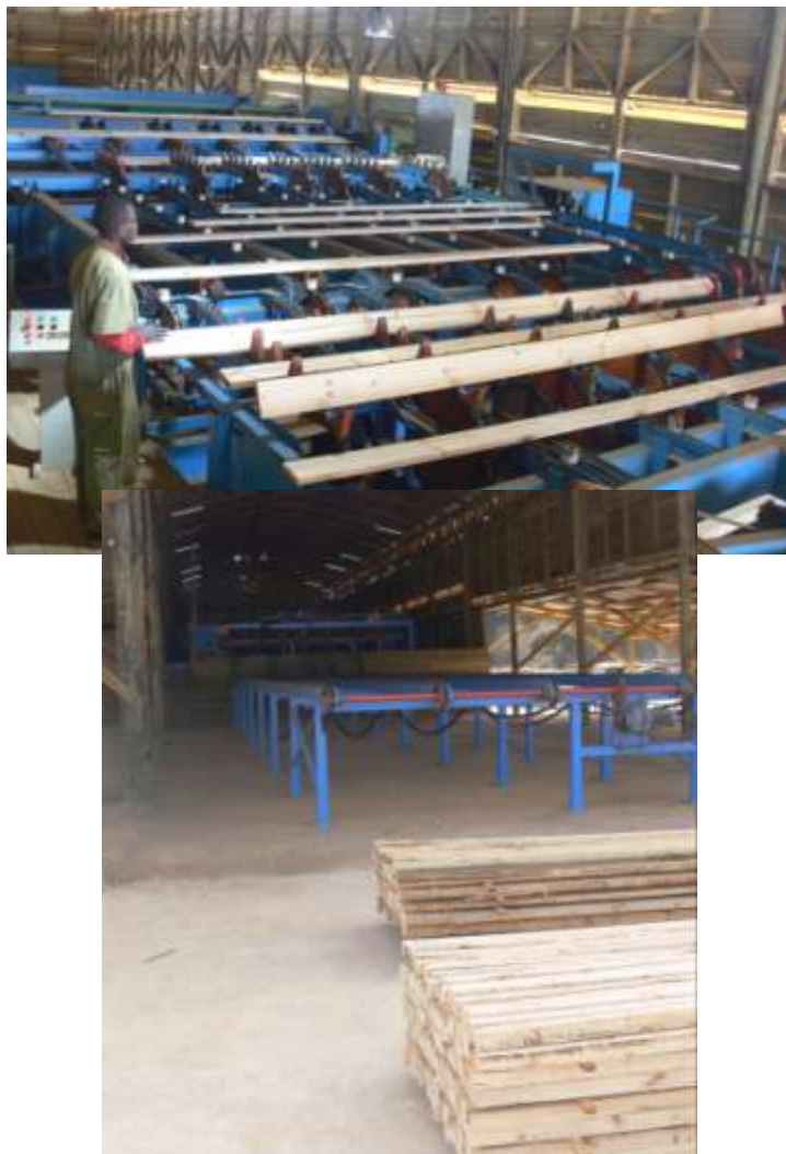
The timber sorting deck and cross saws at the end of the sawmill. This part of the sawmill will also serve the planned new large log sawline at SHI.
