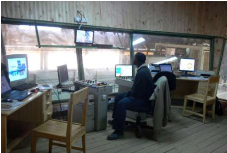
The control room from where the entire sawline is operated.
