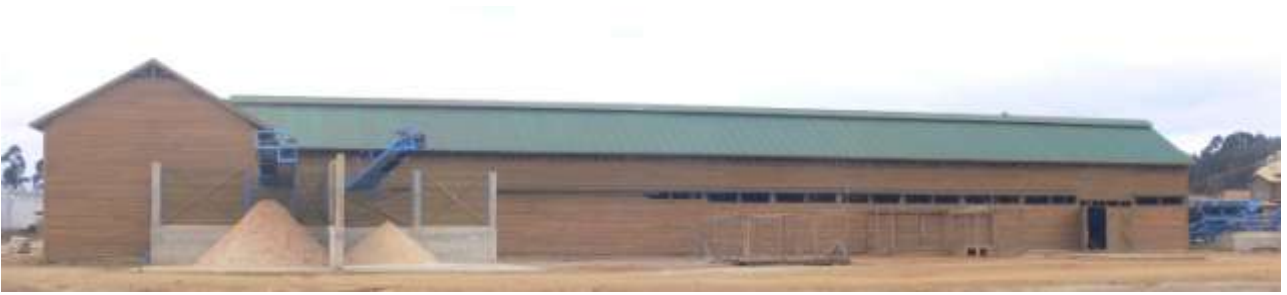
The front of the 100 m long sawmill building. The wood chip and sawdust outfeeds are shown to the left.
