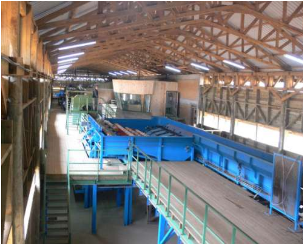
The new 100m long HewSaw sawline, with a potential three shift capacity of 180,000 m3 sawn timber per year. The mill provides high recovery rate for 9-26 cm diameter logs. The new high tech scanner is seen in front of the control room. The guard of the debarking machine is seen to the very right where bark is separated.
