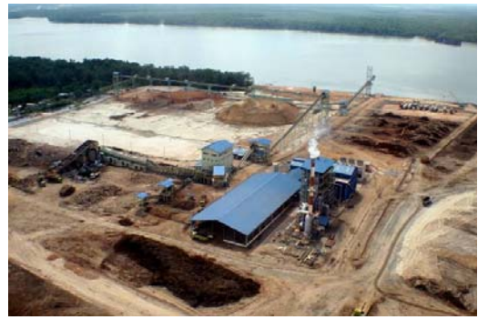
Biomass Boiler and Chip Mill
