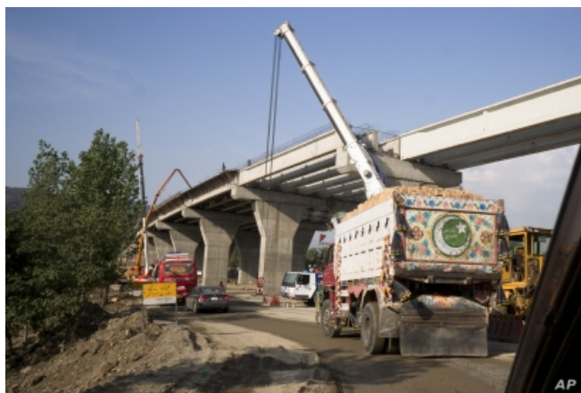
FILE - Construction work is in progress at a new i
