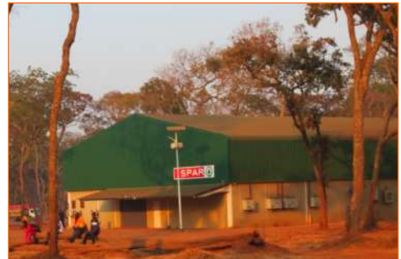
Supermarket and Market Area
