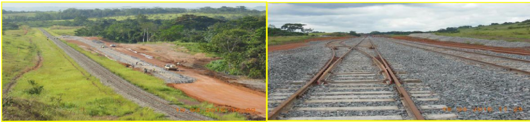
Figure 2 Railway Siding in Franceville
