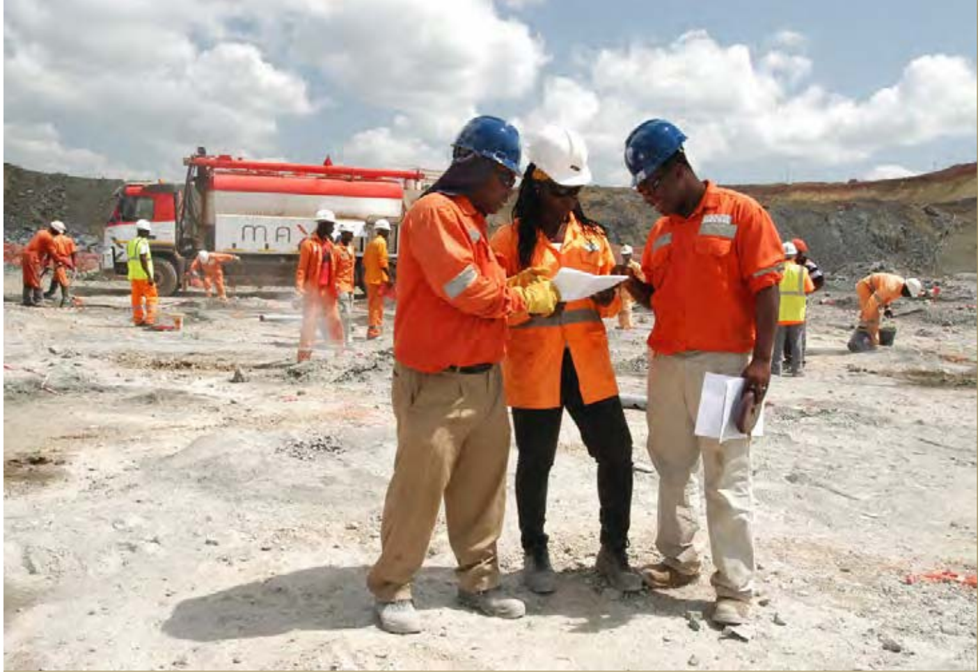
Blast preparation at Tongon's South Zone.
