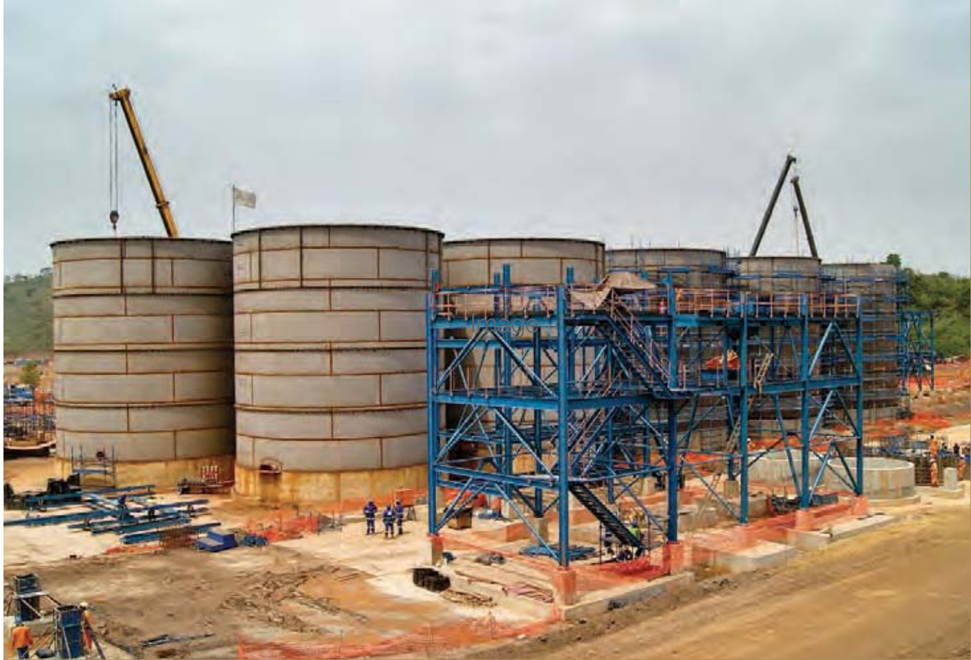
Mill construction at Kibali.
