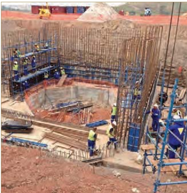
Vertical shaft construction at Kibali.
