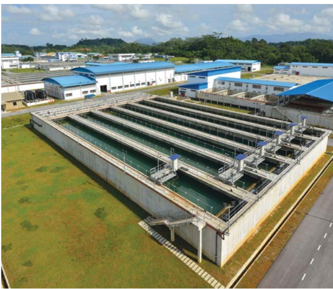
Batu Kintang Water Treatment Plant in Kuching with a treatment capacity of 100,000 m 3 /day
