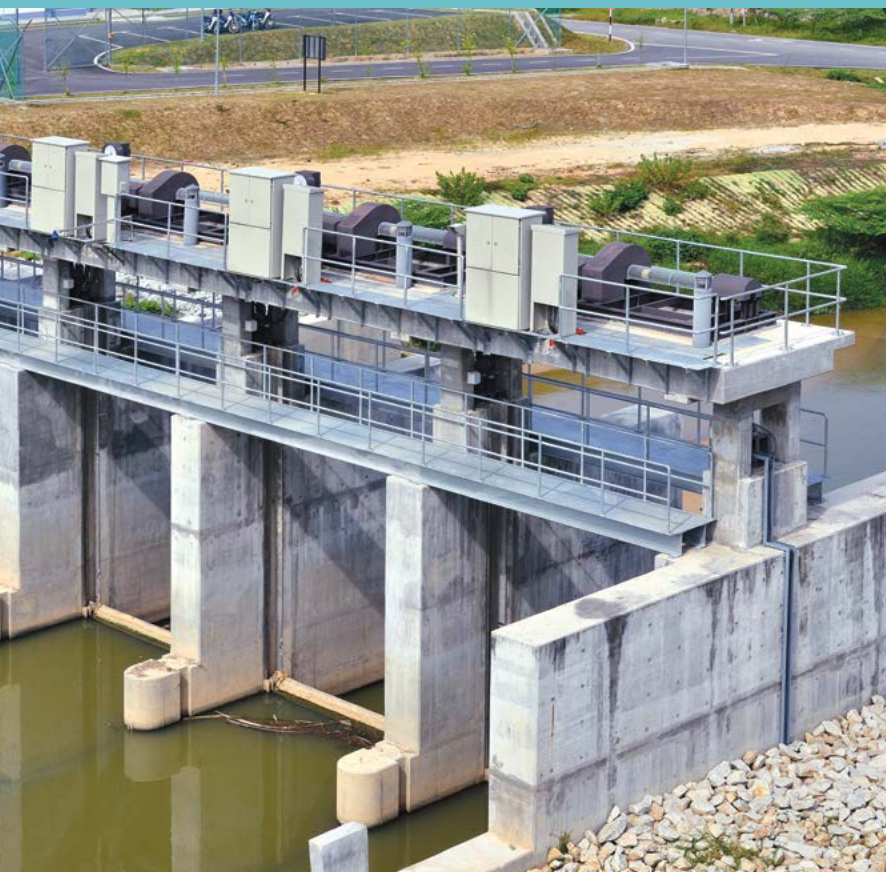
River Gate of KLIA Intake Plant
