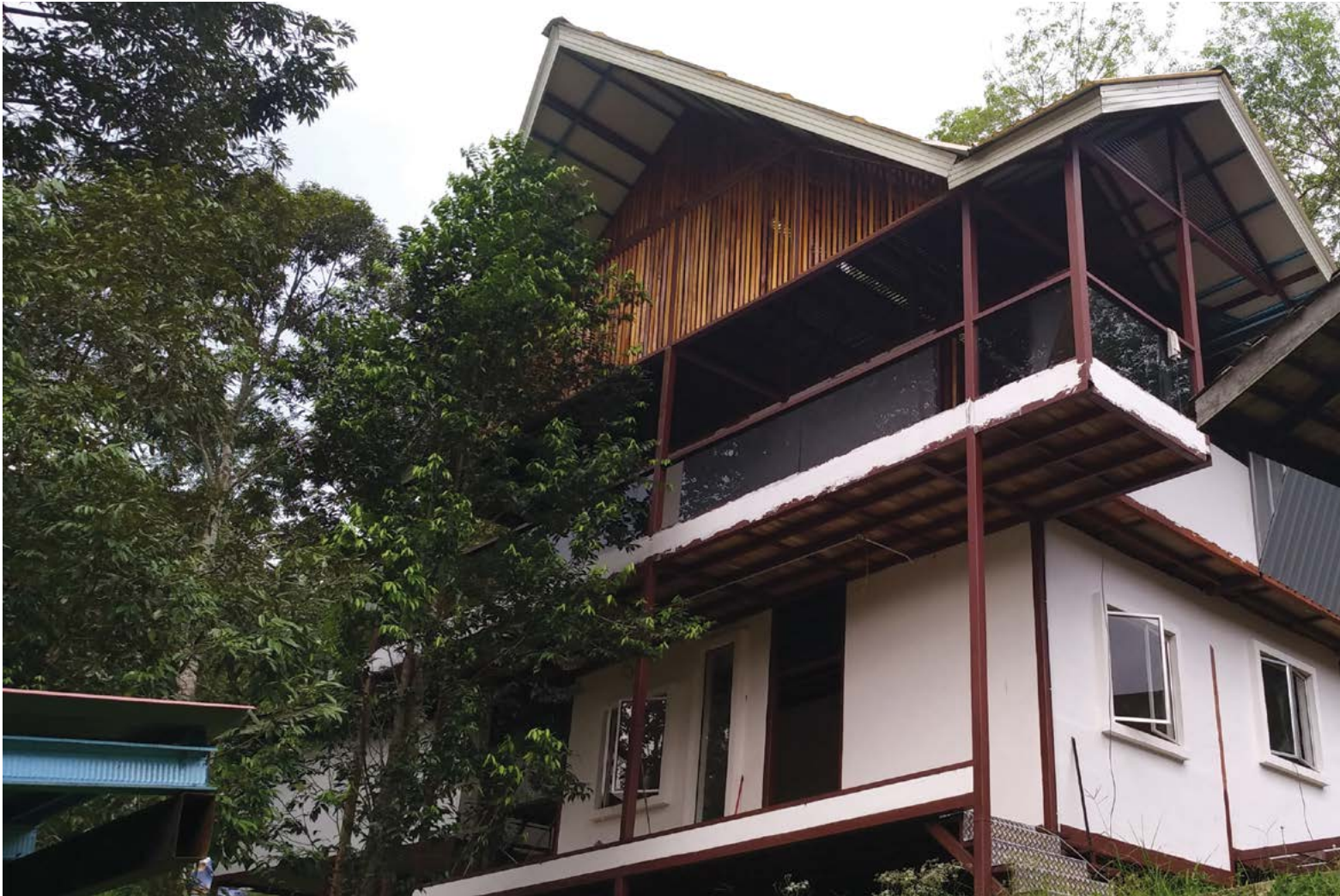
The newly constructed 32-bed dormitory at the Orang Asli Education Centre in Raub, Pahang
