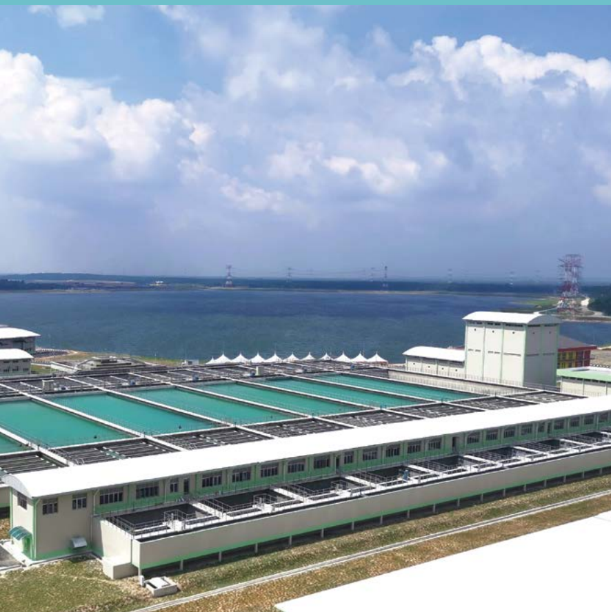
Labohan Dagang Water Treatment Plant
