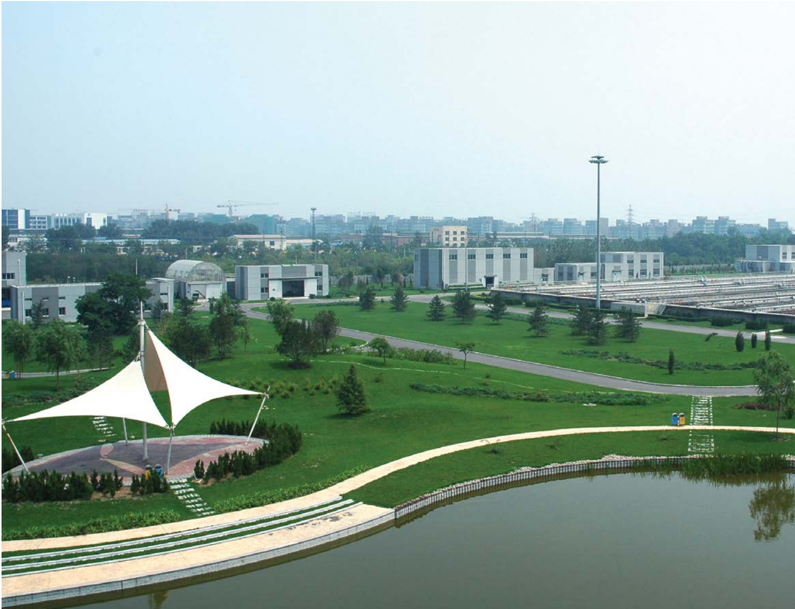
Lugouqiao Sewage Treatment Plant in Beijing is the Group's first sewage treatment plant in China
