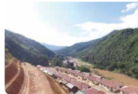
Nam Ou River Level-4 Hydropower Station Resettlement Village
