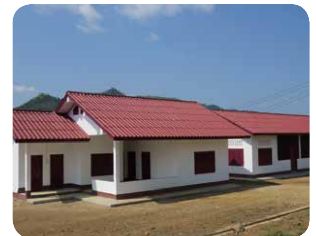
Sop Kinh village administrative office and health center of Level-2 Hydropower Station
