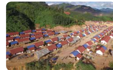
Nam Ou River Level-7 Hydropower Station Resettlement Village
