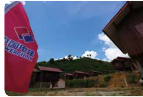
Nam Ou River Level-1 Hydropower Station Resettlement Village
