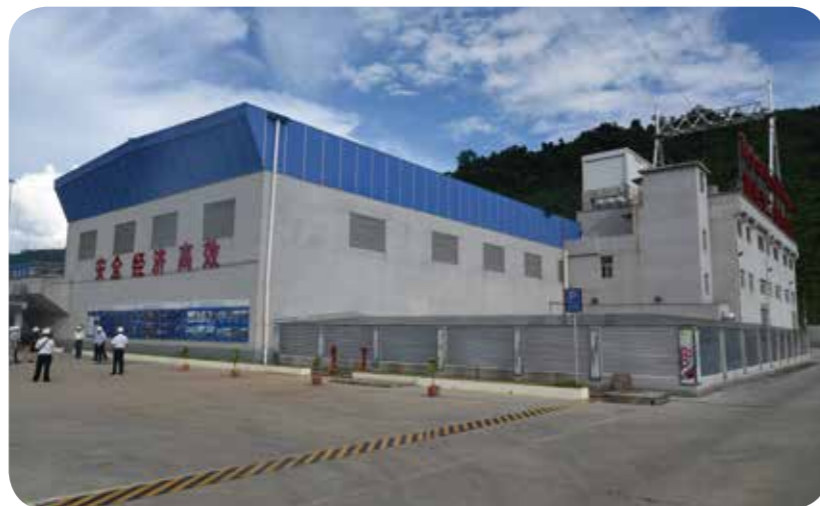
Nam Ou River Level-2 Hydropower Station
