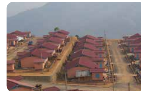
Nam Ou River Level-6 Hydropower Station Resettlement Village
