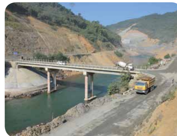
Hat Sa bridge of Level-6 Hydropower Station
