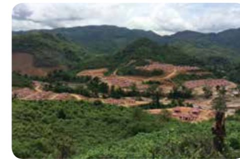
Nam Ou River Level-5 Hydropower Station Resettlement Village
