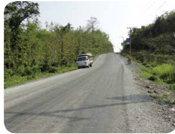
The 8km hardened road of Level-2 Hydropower Station
