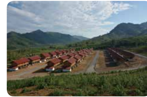
Nam Ou River Level-2 Hydropower Station Resettlement Village
