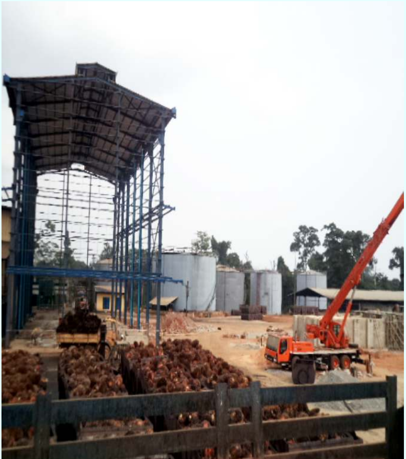
WORK IN PROGRESS IN THE NEW OIL MILL
