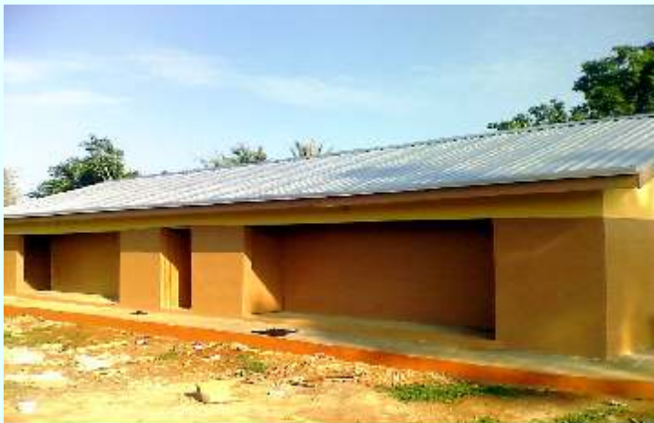
FIRST SANITARY PAVILION AT AMADAGBAYO BUILT BY OKOMU
