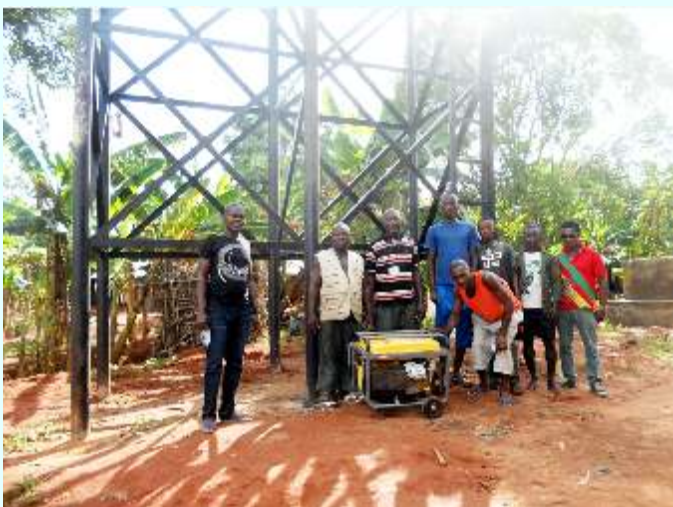
CONSTRUCTION OF BORE HOLE AND WATER STORAGE SYSTEM AT MARIOGHIONBA
