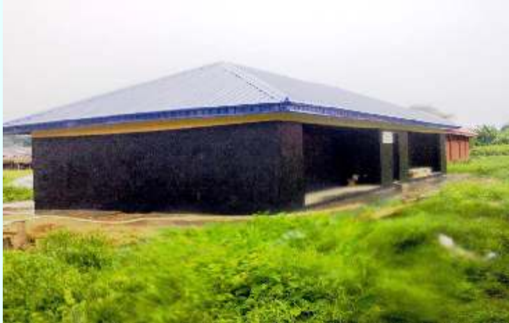
SANITARY PAVILION AT INIKOROGHA PRIMARY SCHOOL BUILT BY OKOMU
