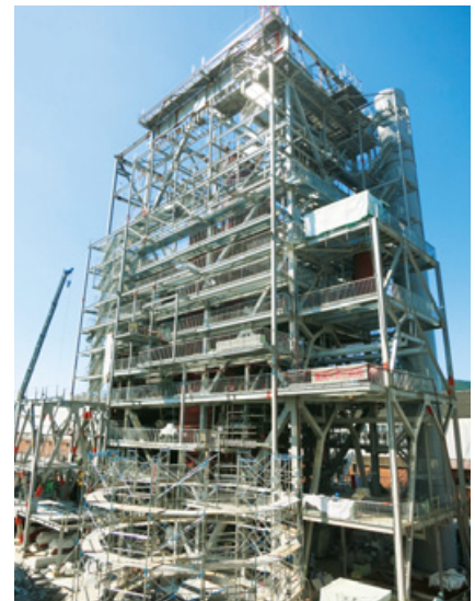
Biomass boiler under construction (Oji Green Energy Nichinan/Nichinan, Miyazaki)
