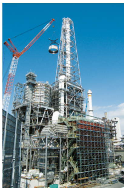
Oji Materia Fuji Mill's biomass boiler under construction (Shizuoka)
