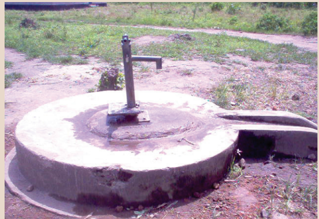
Manual pump well built at Mbasa primary school. © Oakland Institute
