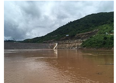
Nam Ou 3 station part of phase II of the Nam Ou cascade hydropower project
