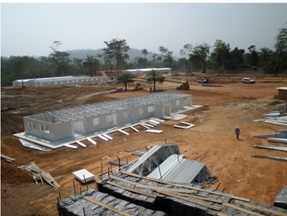
Kokoya New Camp Construction
