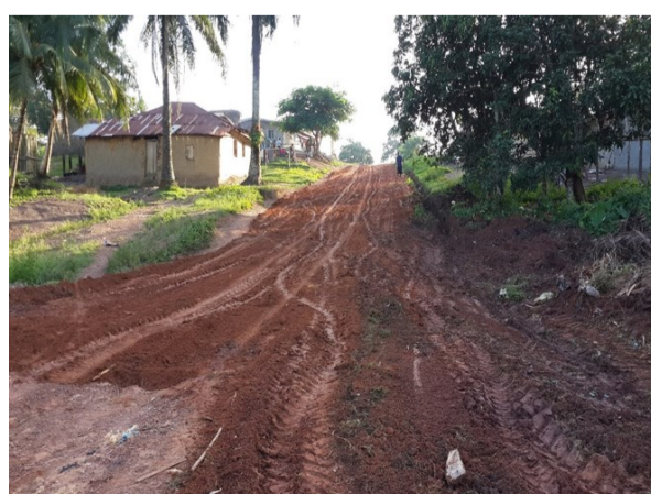
Rehabilitation of roads
