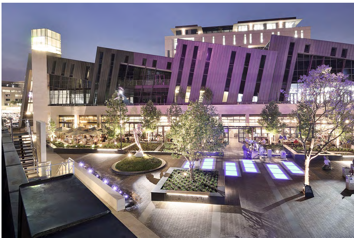
PIC Office building. Source: https://www.linkedin.com/company/public-investment-corporation/?originalSubdomain=za .
