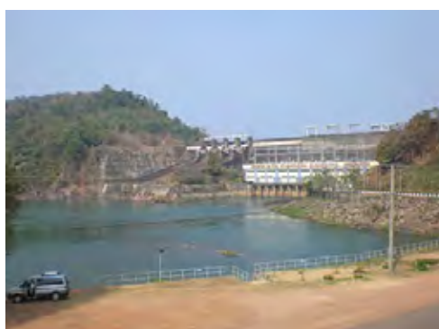
NN1 Hydropower Station
