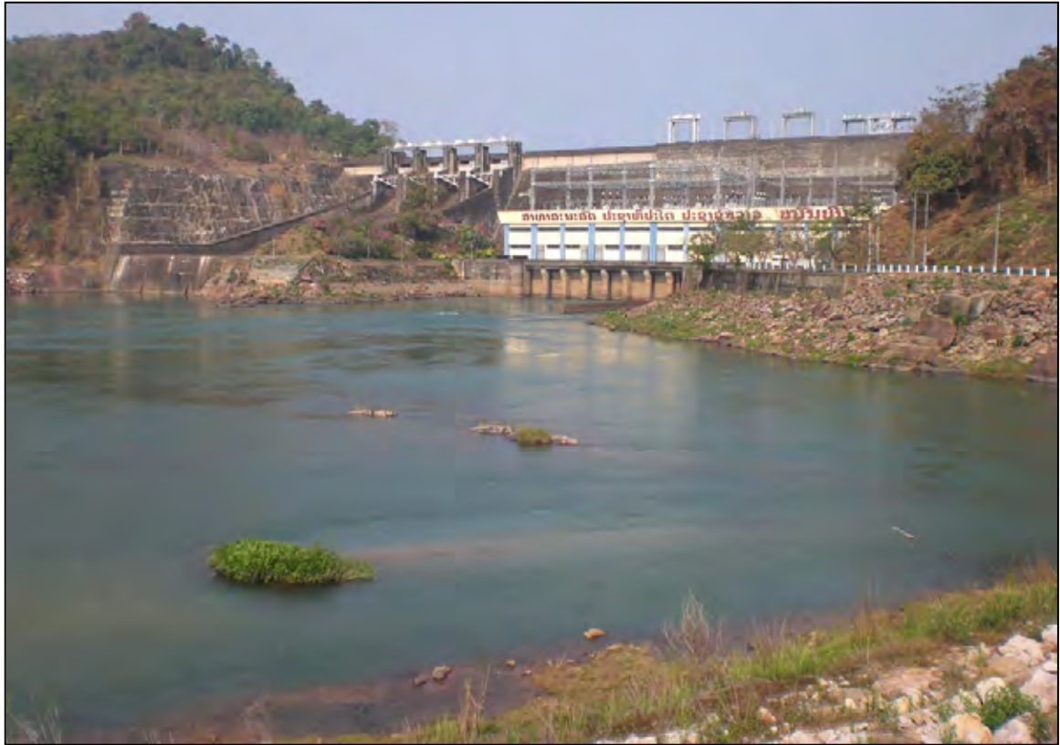
Nam Ngum 1 Dam and Power Station
