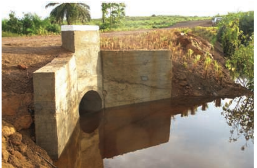
One of the rehabilitated culverts
