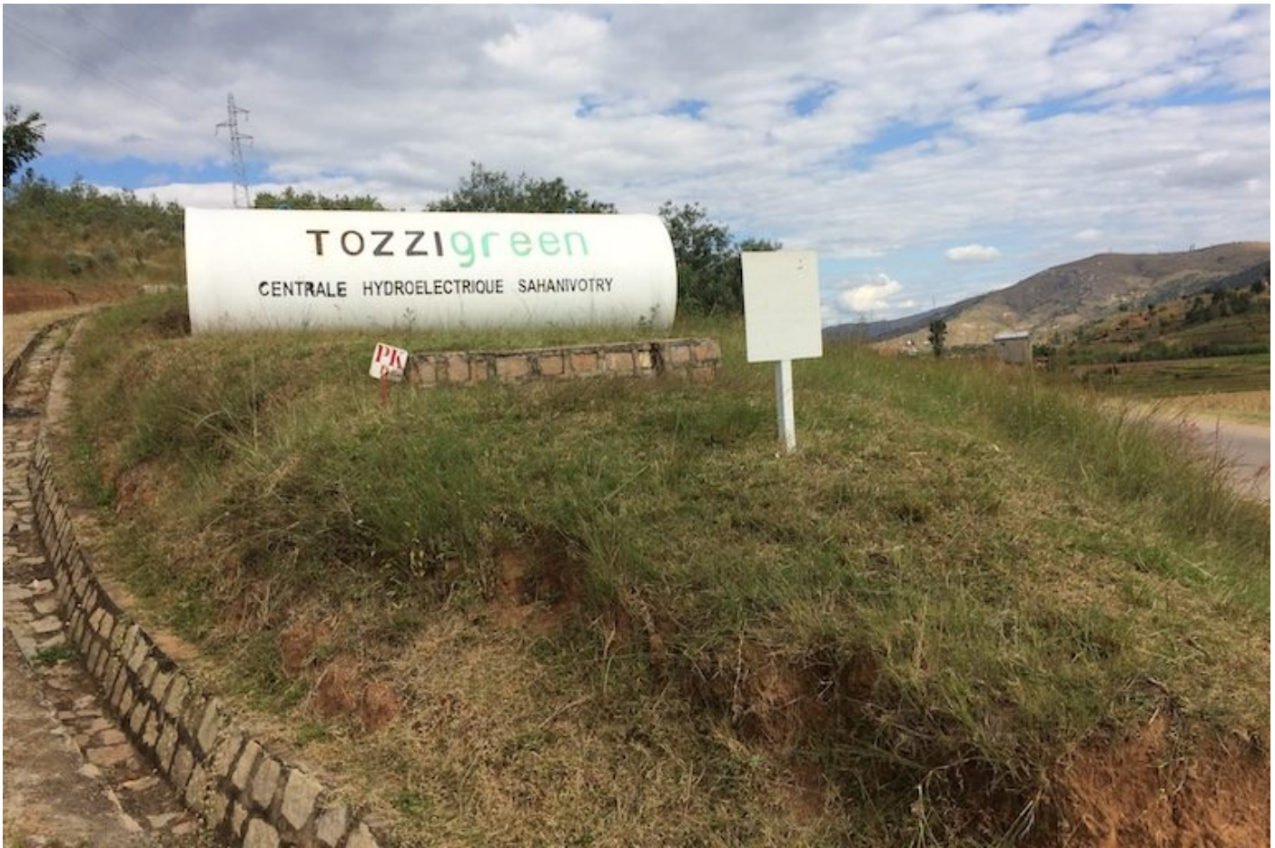
Tozzi Green already has a power plant near the village of Sahanivotry, and the proposed new dam, several kilometers downriver, would allow it to double its electricity output. Image by Edward Carver for Mongabay.
