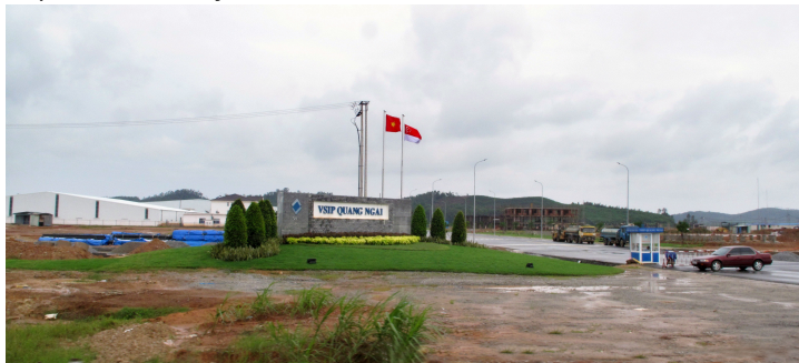
Several factories under construction in VSIP Quang Ngai
