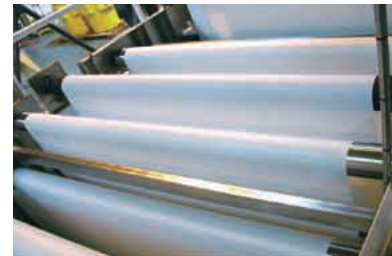
Using membranes makes the water treatment process less expensive and safer.
