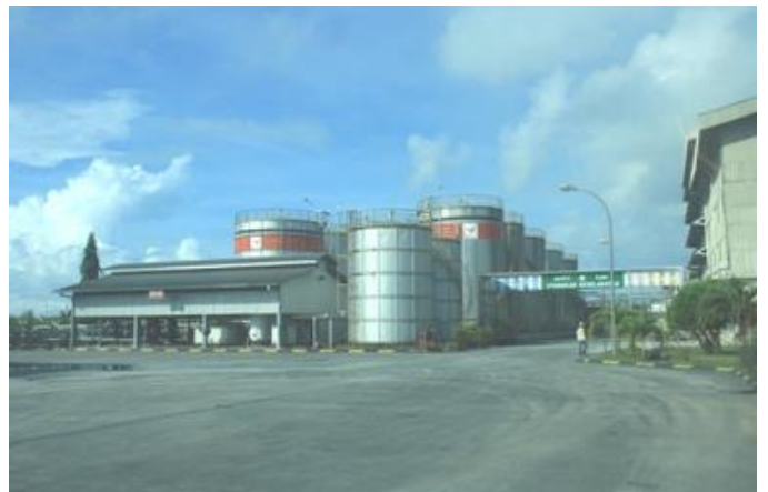
Figure 154: Storage tank next to refinery facilities
