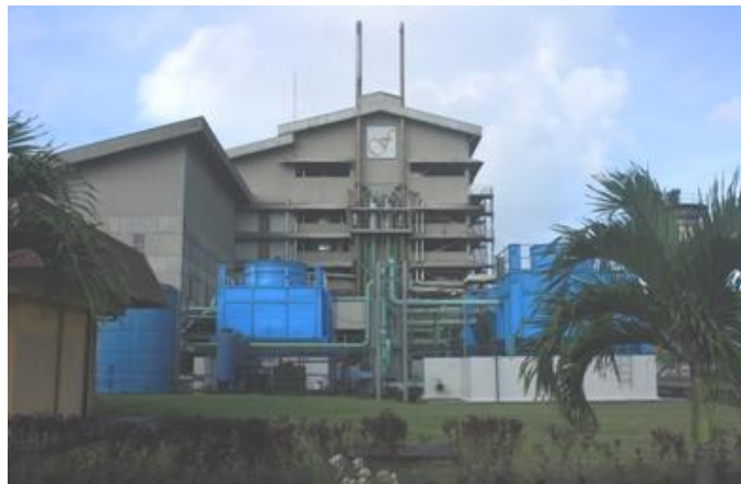
Figure 153: Refinery at Sahabat estate
