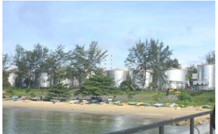
Figure 158: Storage tank facility located next to jetty
