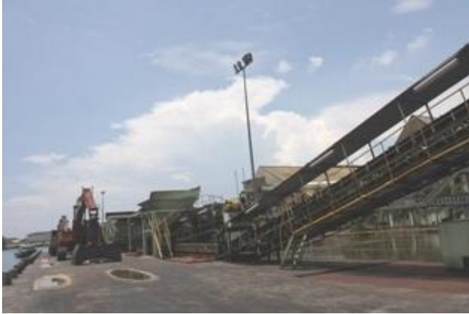
Figure 169: Port and conveyor
