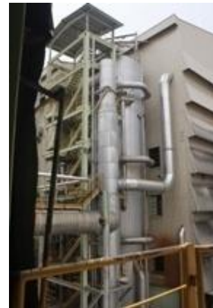
Figure 172: Vertical continuous crystalliser – MSM only
