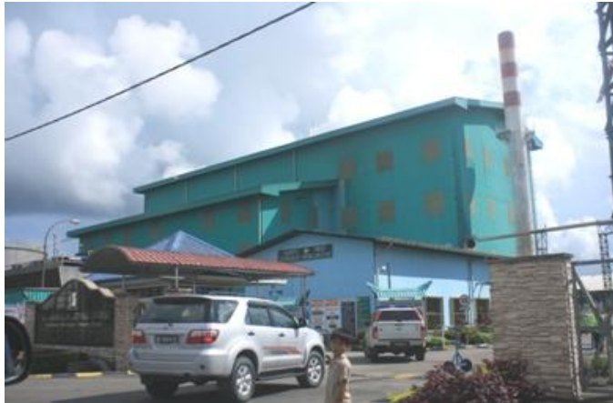
Figure 155: Sahabat biomass power plant
