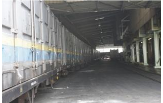
Figure 174: Railway in MSM facility
