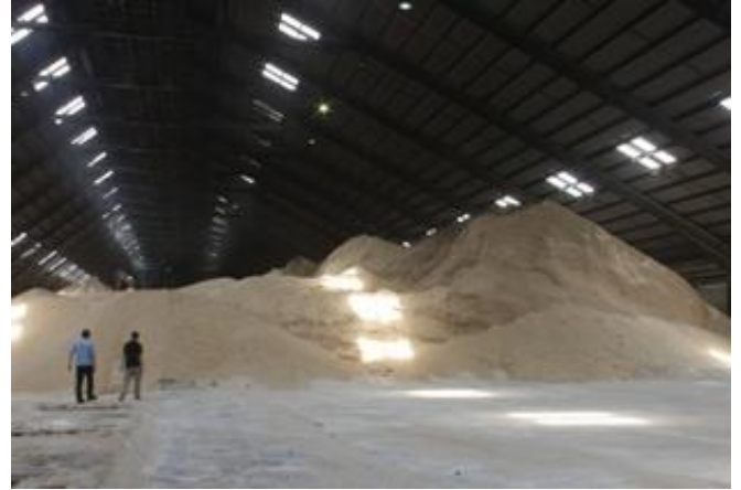
Figure 170: Raw sugar warehouse
