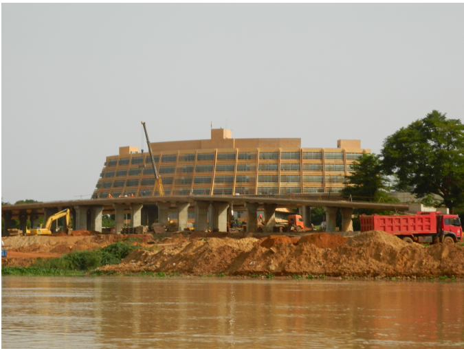
Flyover under construction near the Niger River in downtown Niamey, Niger.
