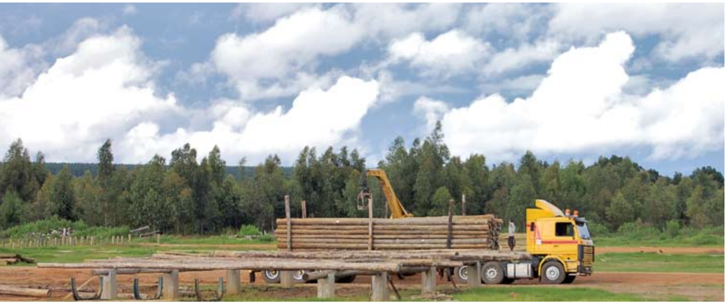
Loading transmission poles
