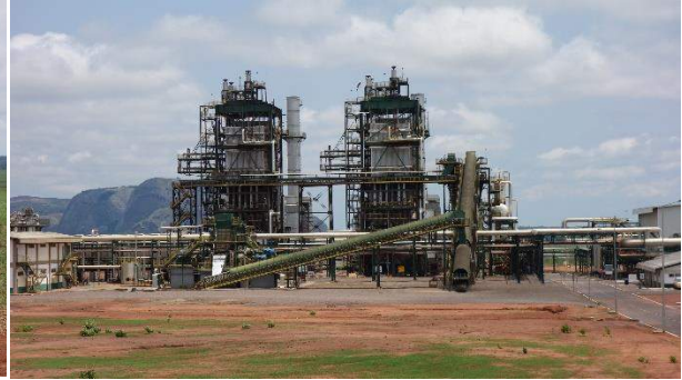
Biocom Sugar / Ethanol plant
