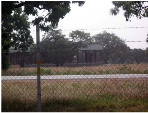
ITFC Packhouse under construction
