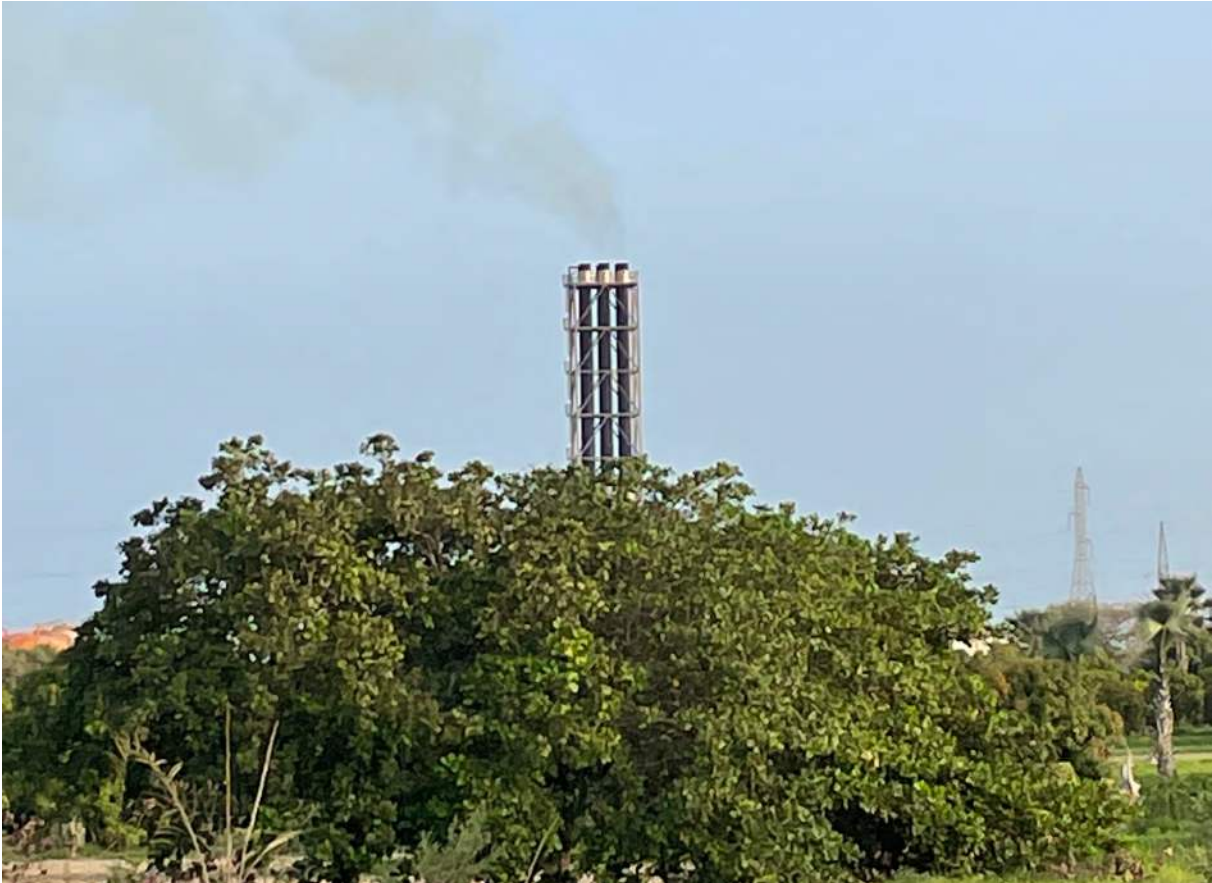
Tobene power plant with emissions, close to the wind farm
