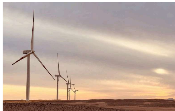
The 250-MW West Bakr wind farm in Egypt. Image by Lekela.
