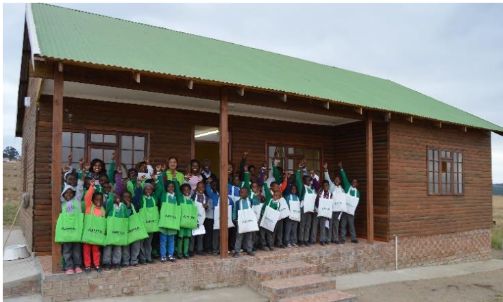
Vriesland Primary School Kitchen
