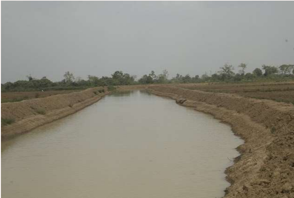
Part of the irrigation channel that supplying water to the rice field
