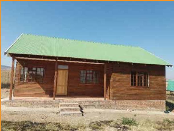
Vriesland Primary School Kitchen
