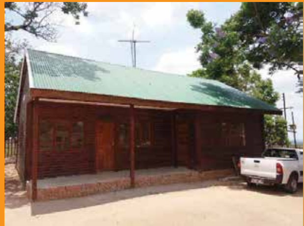
Marongwane Primary School – Kitchen
