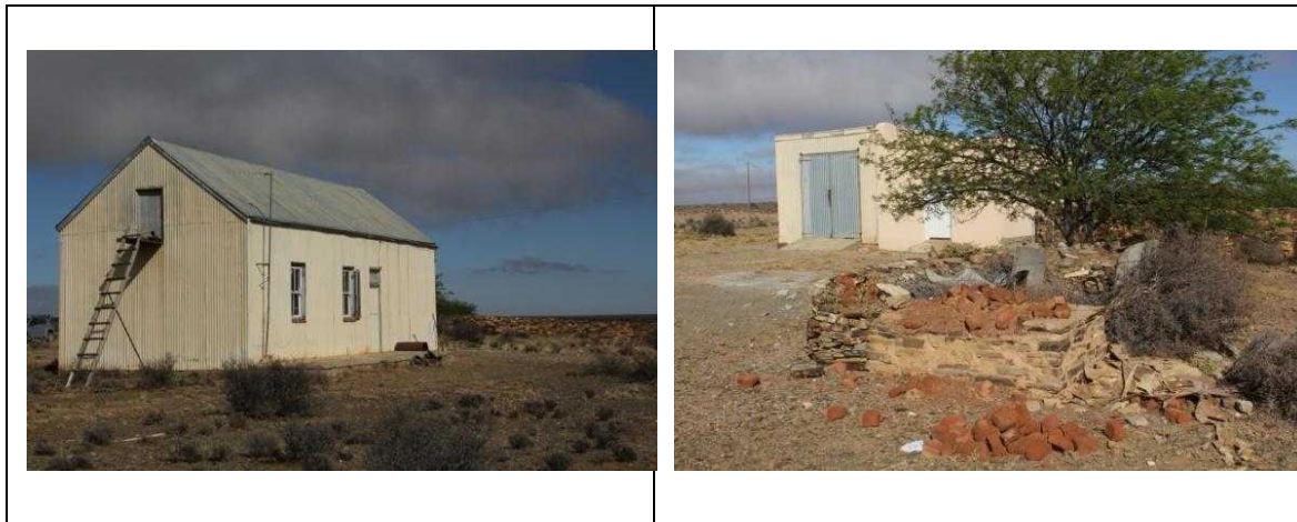
Figure 95: Views of the farmstead
