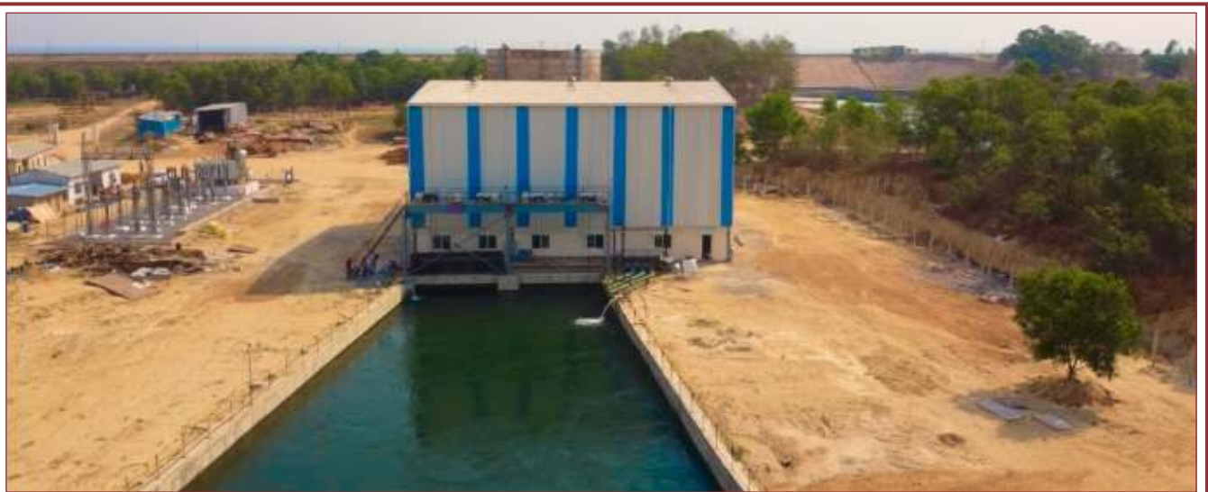
IREDA funded 9.00 MW Small Hydro Project of M/s. Kakatiya Industries Private Limited, located at Hirakud Dam on Mahanadi River near Village - Rengali, Taluk- Attabira, District- Baragarh, Odisha.
