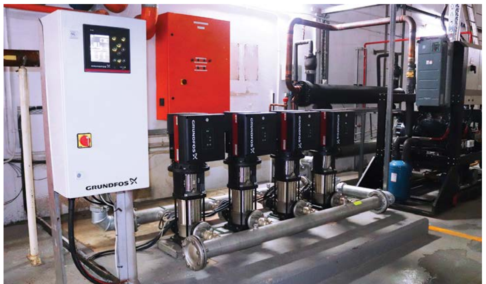
The Grundfos hydro MPC-E booster pump set with four 7,5 kW motors and CIM 500 control system.
