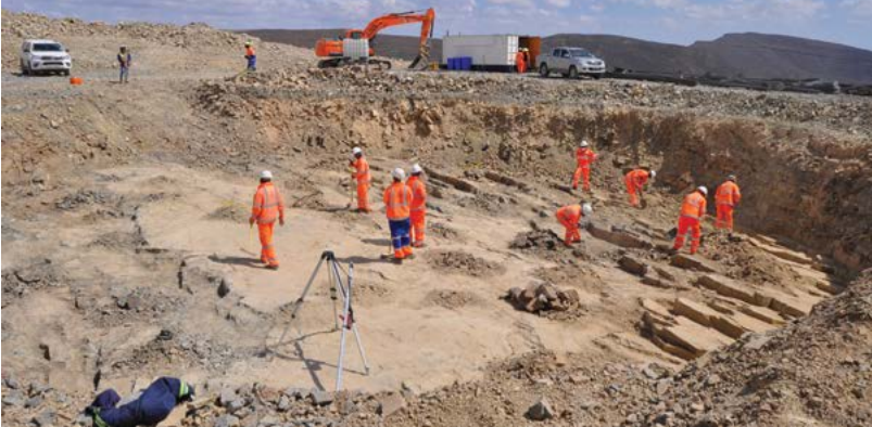
Cleaning of a foundation underway at Roggeveld Wind Farm.
