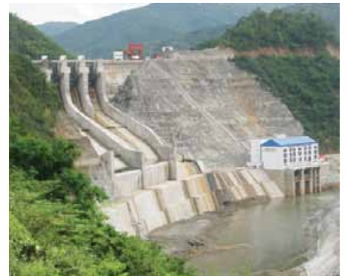
A view of Nam Khan 2 hydropower project in Luang Prabang.
