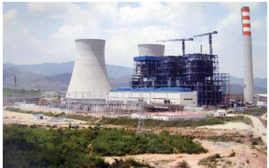
The Hongsa Mine-Mouth Power Project is under construction in Xayaboury province.
