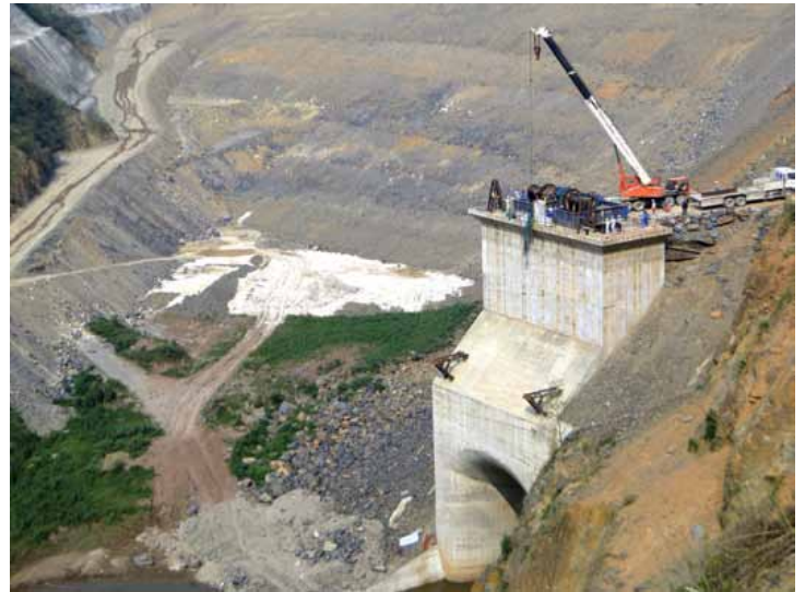
A view of the diversion tunnel of Nam Khan 2 hydropower project.
