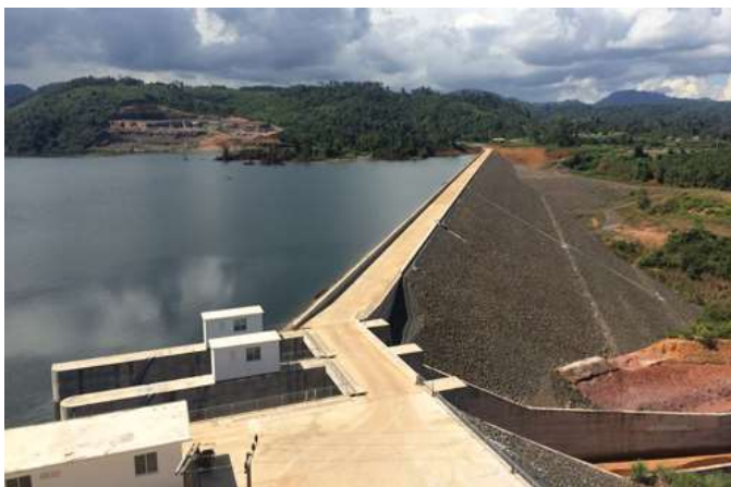
Completion image. [Photo / cggc.cc]
