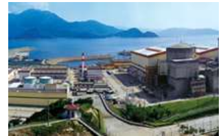
Dayawan Nuclear Power Plant (China)
