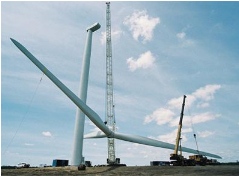
Figure 3.3: A wind turbine in the process of being erected 17
