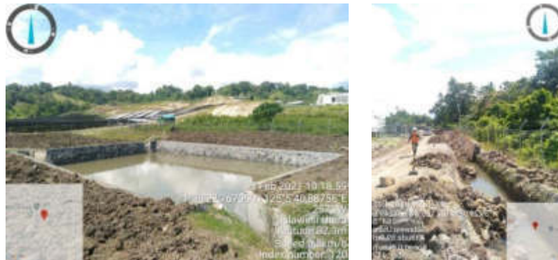
Figure 6 – Drainage and settlement pond construction at the site.
