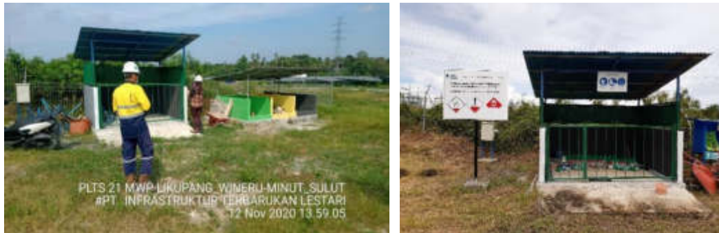
Figure 18 – Assessment from local Government and improvement of the building after the assessment
