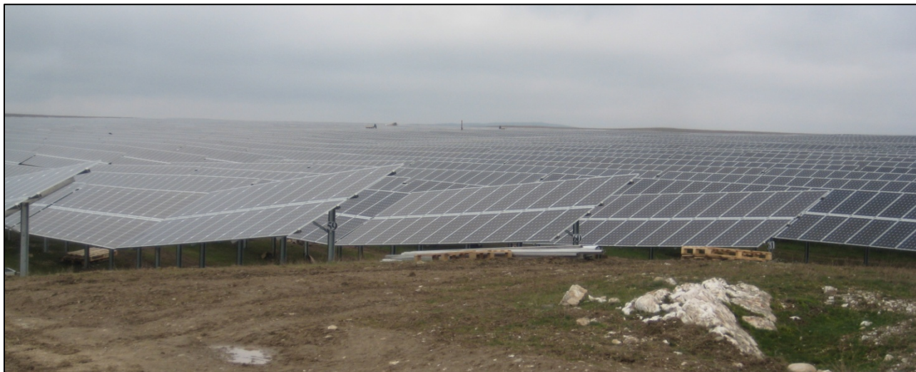
Photo 1 Sunlight photos knock off electrons in photovoltaic panels that create electric current.
