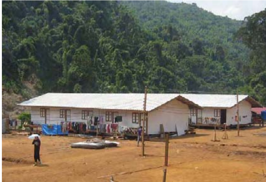
Figure 3: Work Camp at Power House (2007).
