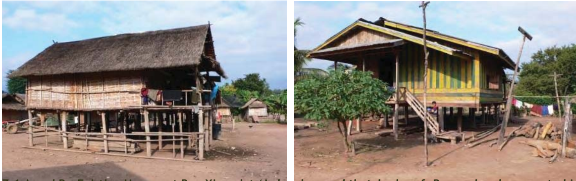
Figure 7-1 A and B: Existing Houses at Ban Xiengdet (A: bamboo and thatched roof; B: wood and corrugated iron roof)
