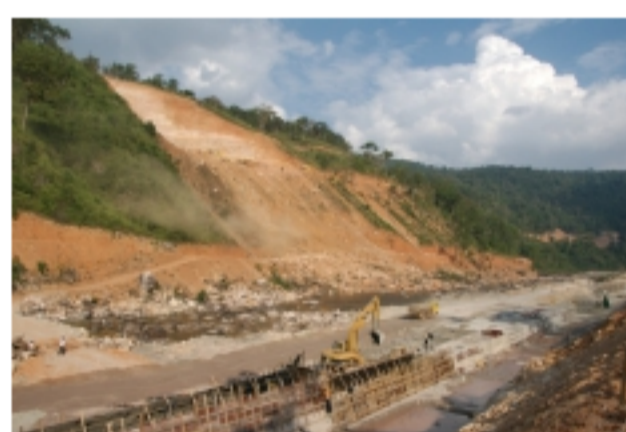
Construction work at the Kamchay Dam site - 2008 © Marcus Rhinelander
